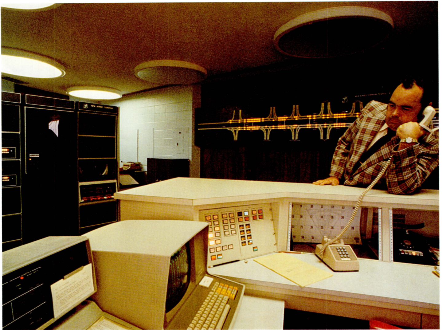
Traffic control of a busy, forty-mile section of the New Jersey Turnpike is accomplished through use of a Digital PDP-11 computer. Sensors embedded in the highway surface transmit traffic information to a control center where the data is translated into a visual display on a large illuminated map. If the system identifies unusual traffic conditions, it can automatically activate warning or directional signs to alert motorists.
